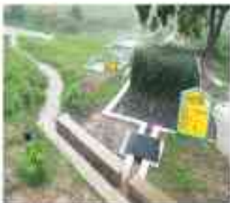
Figure 8.1: Horizontal filtration system
